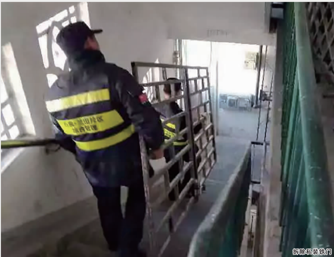
拆除私装铁门
