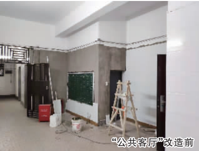
“公共客厅”改造前
